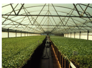
Figure 11. Galvanized steel tubing is often used in constructing greenhouses to be used for transplant production. Steel tubing facilitates maximum light transmittance.
