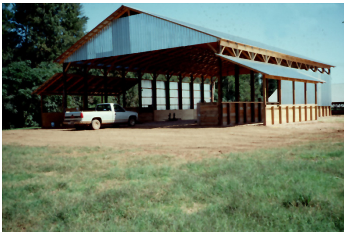
Example of a litter storage and mortality composting structure.
