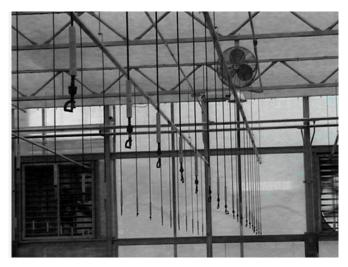
similar in terms of the sprinklers required. Overhead lines require rigid pipe, and can be set up to move from one bench or side of the greenhouse to the next. Overhead lines are usually in greenhouses or shade structures to keep them out of the way of carts and people. In ground or above ground lines are typically found on outside production beds and should also be placed carefully to keep them out of traffic patterns.
