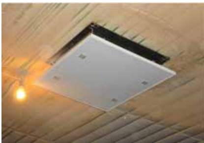
Figure 6. With an insulated attic, the air is warmer than outside air. Using the air allows higher ventilation rates to be used without increasing fuel usage. These increased ventilation rates will help maintain relative humidity between 50 and 70 percent.
