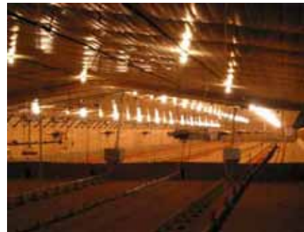
Figure 5. Air entering through the inlets is directed along the ceiling. This allows the air to warm up to brooding temperature before coming into contact with the chicks. This also increases the moisture holding capacity of the air so that when the warm air does fall down to chick level it will pick up and hold more moisture from the litter helping to maintain litter conditions in the house.
