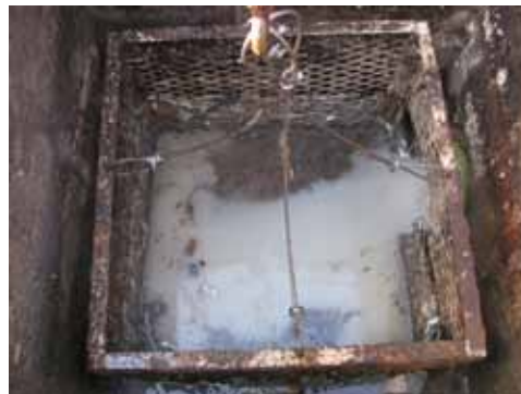
Figure 8. A manually operated basket screen is used to capture grit prior to the wastewater treatment system at a shell egg processing plant. If cleaned on a consistent, periodic basis, static basket screens can be efficient grit recovery devices.
