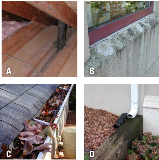
Figure 8. Sources of moisture around and in structures include, but are not limited to: (A) collection of water in attics from leaky pipe penetrations on the roof, (B) collection of water behind improperly installed siding around windows (note growth of lichens, indicating excessive moisture accumulation), (C) leaf-clogged gutters, and (D) downspout exhaust too close to the structure.
