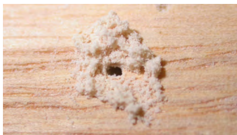
True powderpost beetle frass and exit hole in an oak shelf
