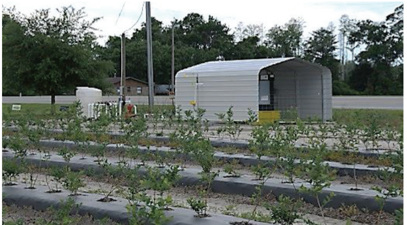
Figure 4. A shed constructed over the well head, pump motor, and electrical controllers.
