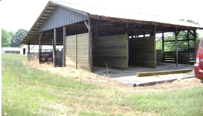
Renovating an existing structure
